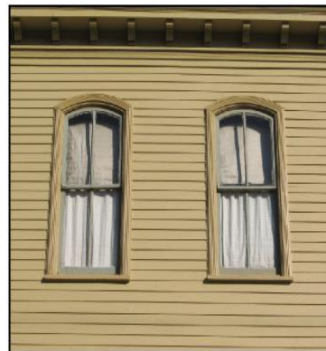
Original two-over-two wood sash, arched windows.
