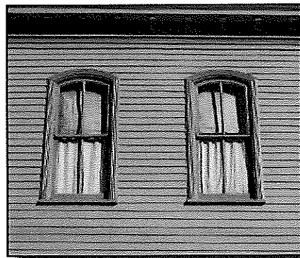
Original two-over-two wood sash, arched windows.
