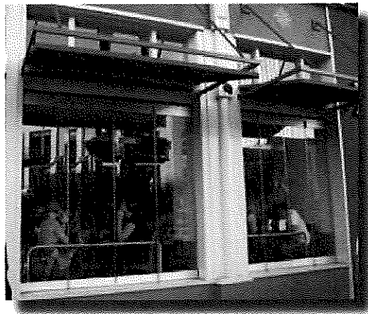
Side-hinged retractable windows on infill building.
