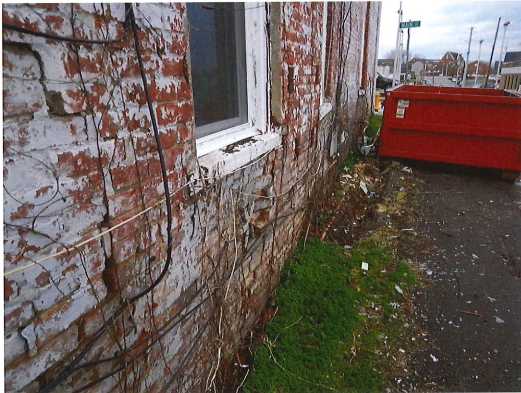
Photo No. 20: Displaced brick masonry on the east side of the building.
