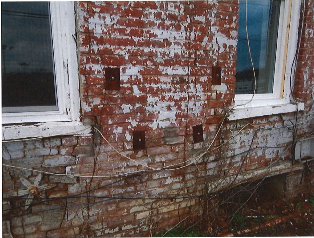
Photo No. 19: Supplemental bracing for displaced brick masonry on the east side of the building.
