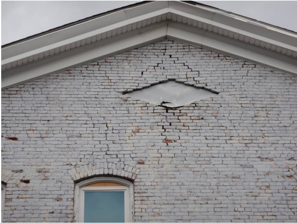
Photo No. 21: Missing mortar and mortar joint cracking on the south side of the building.
