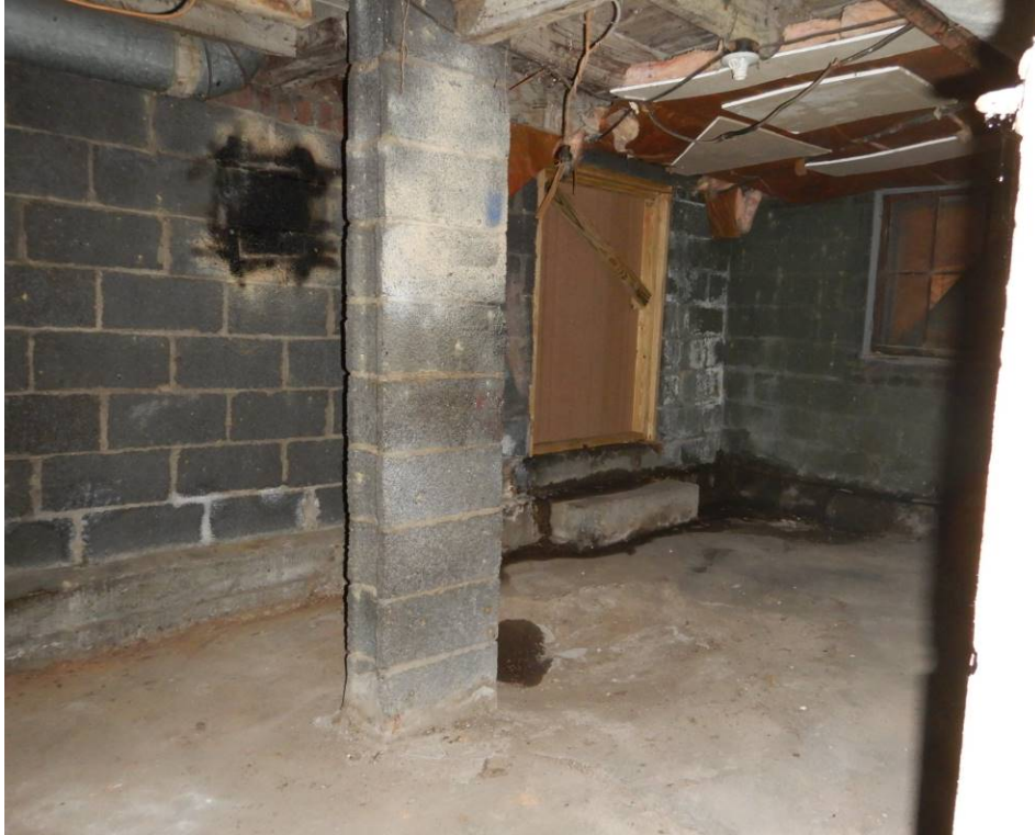
Photo No. 50: Water staining and efflorescence along the base of the foundation wall in the basement.
