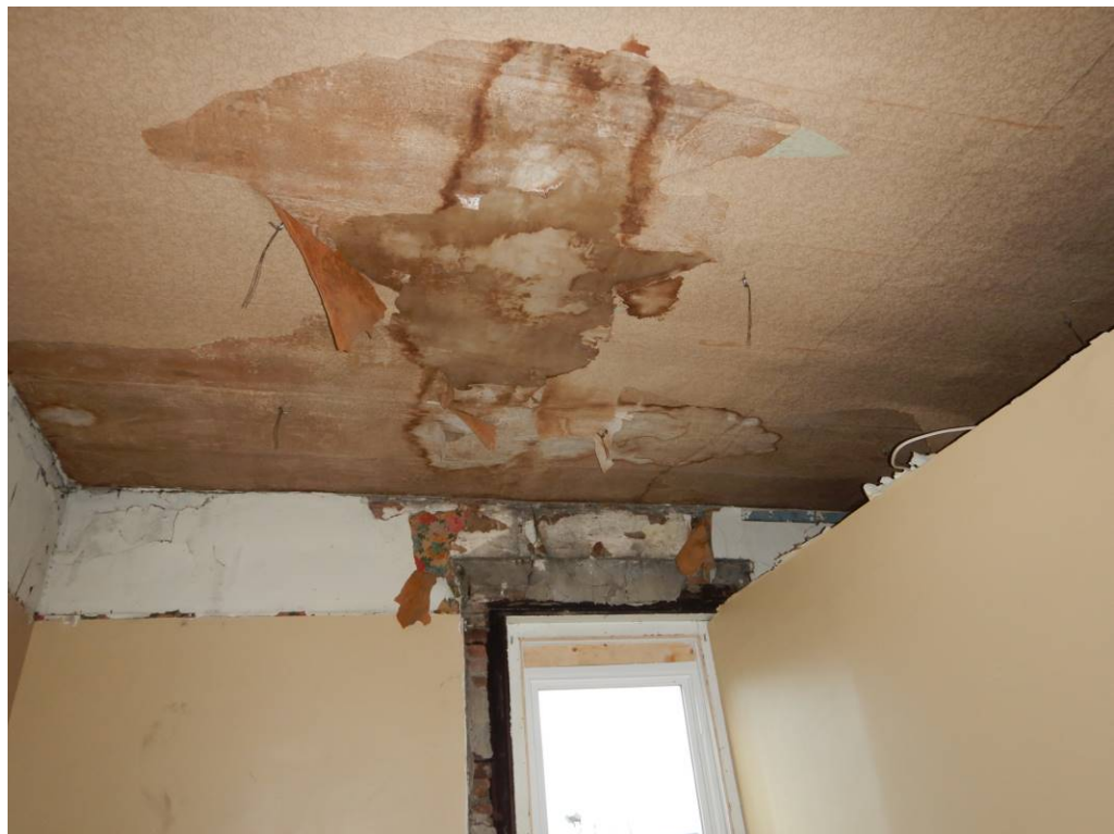
Photo No. 48: Water staining on a ceiling on the upper floor.
