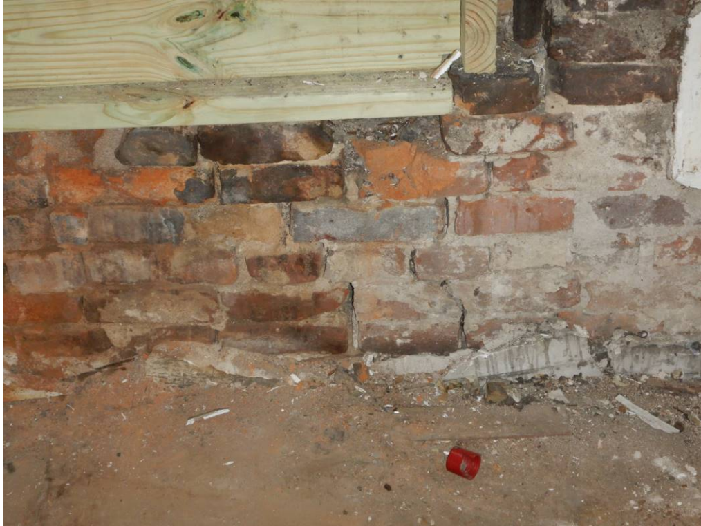
Photo No. 46: Cracked masonry beneath a replacement window installation on the upper floor.
