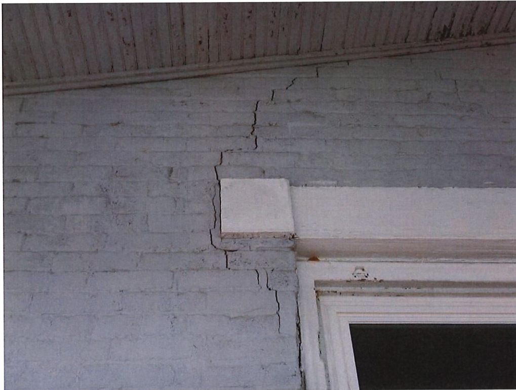
Photo No. 10: Missing mortar and mortar joint cracking on the north side of the building.
