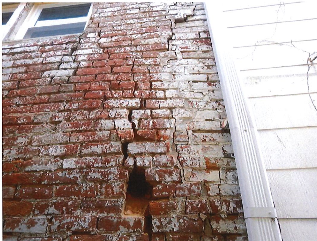
Photo No. 26: Missing mortar and displaced masonry on the west side of the building.
