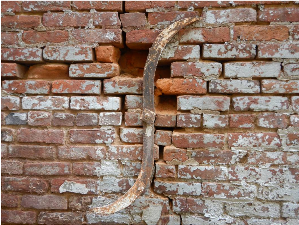
Photo No. 29: Missing mortar and bricks on the west side of the building.
