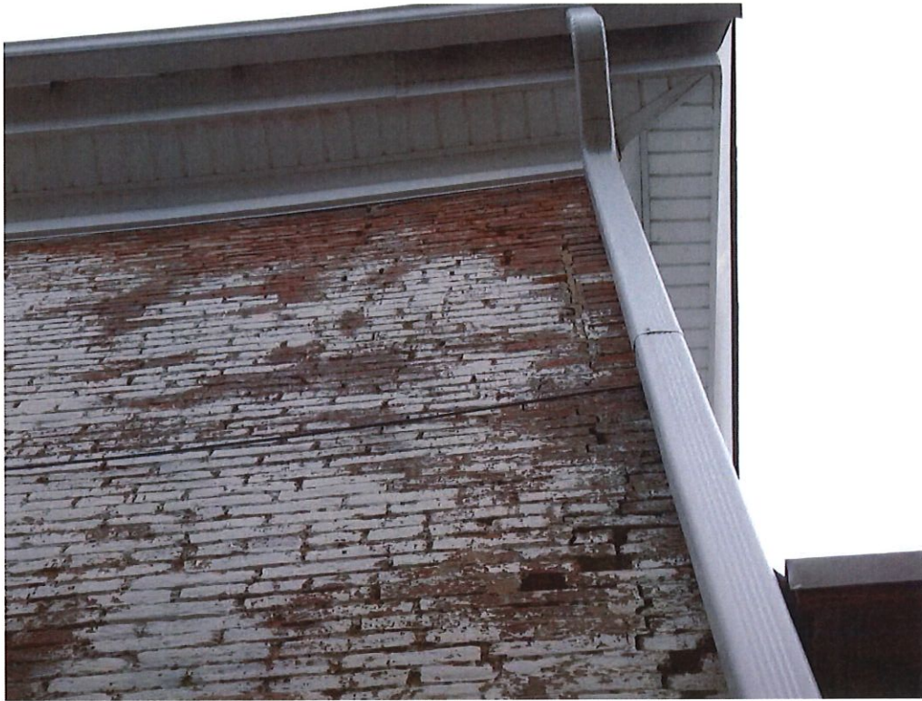
Photo No. 25: Missing mortar and mortar joint cracking on the west side of the building.
