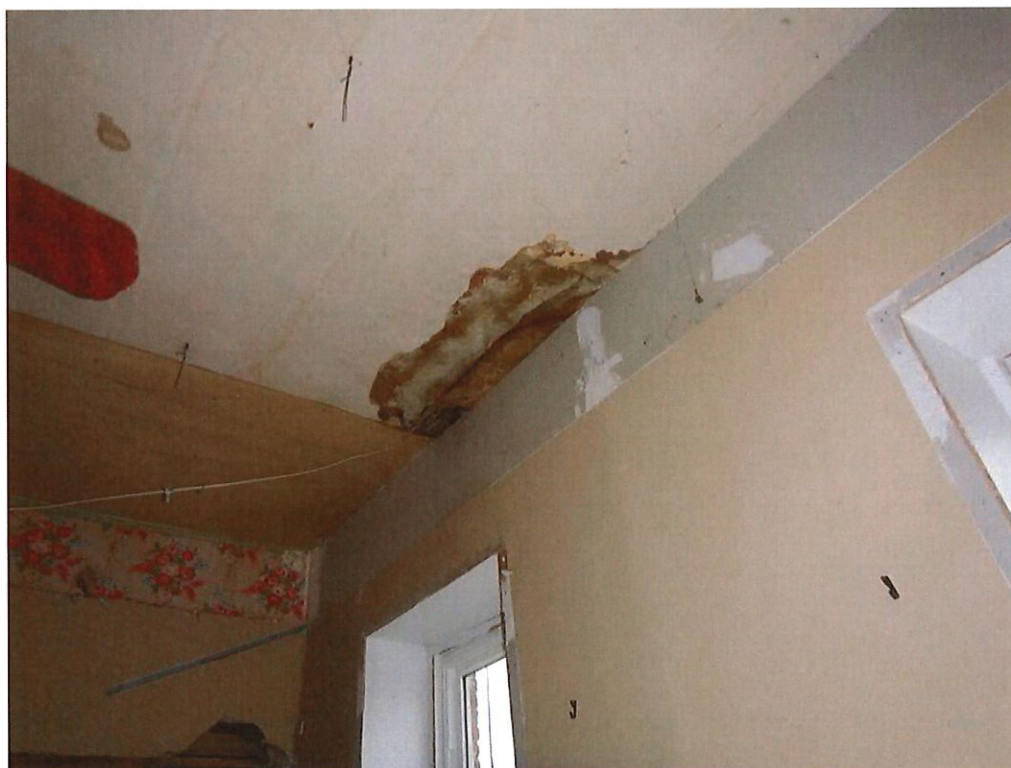
Photo No. 38: Water staining in the ceiling adjacent to a main floor exterior wall.
