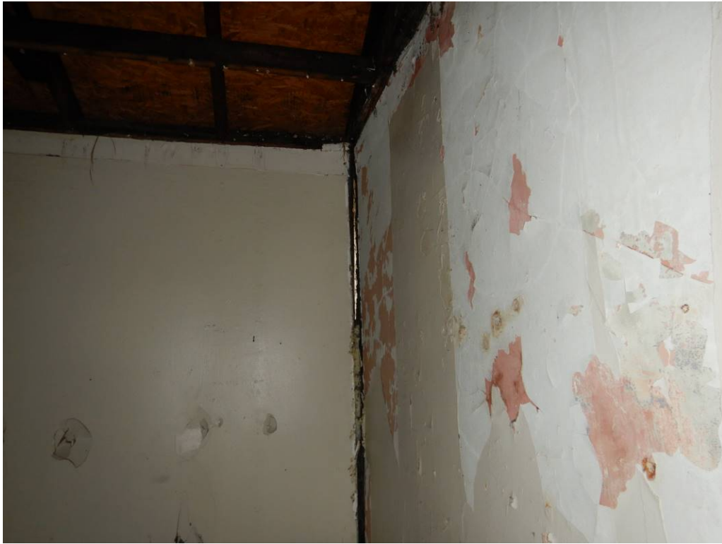
Photo No. 41: Gap between the rear addition and the main structure.
