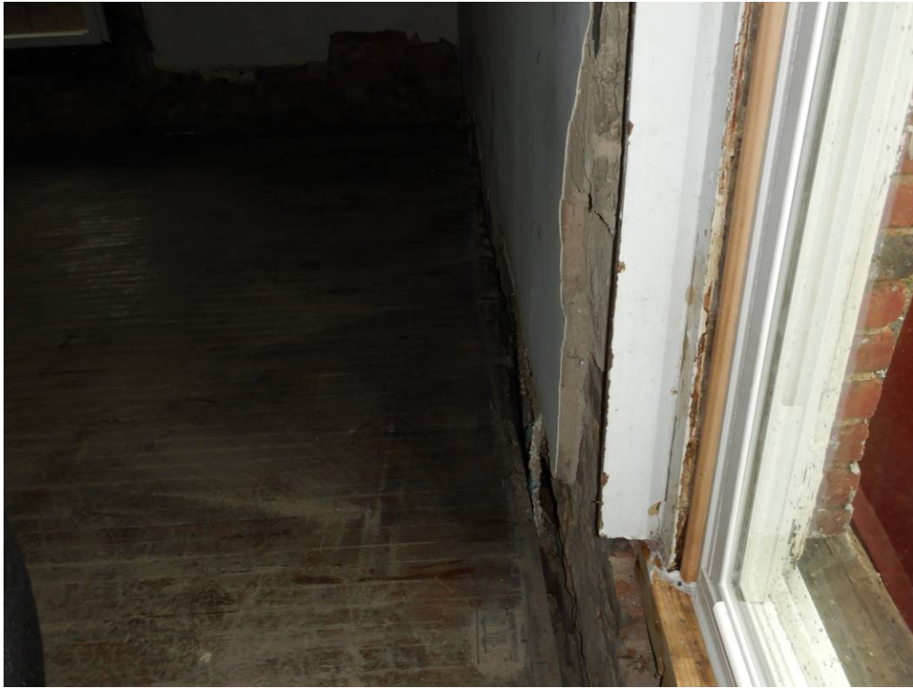
Photo No. 37: Gap between the floor covering and the masonry wall on the main floor.
