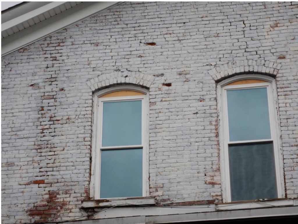
Photo No. 22: Missing mortar and mortar joint cracking on the south side of the building.
