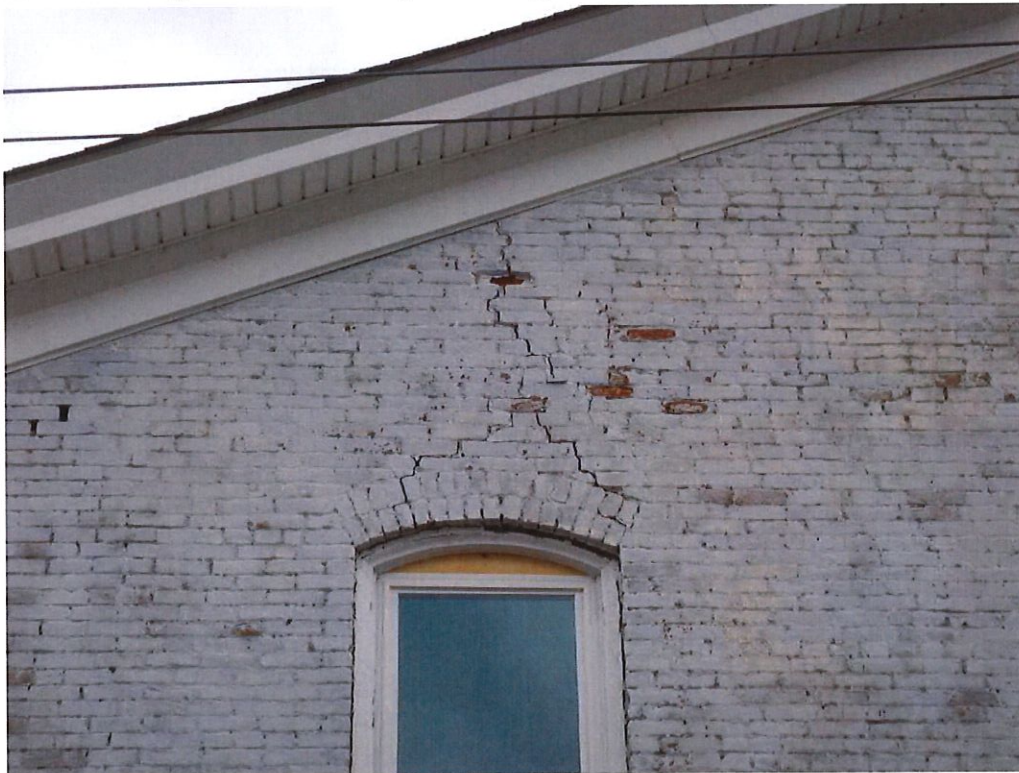
Photo No. 8: Missing mortar and mortar joint cracking on the north side of the building.
