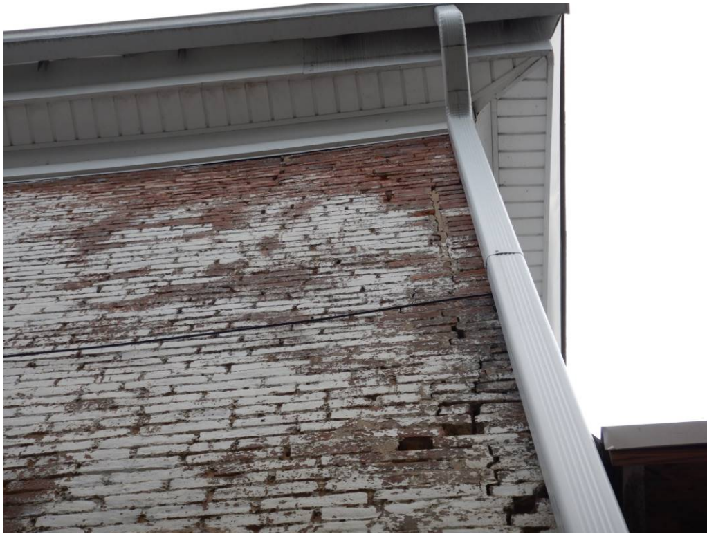
Photo No. 25: Missing mortar and mortar joint cracking on the west side of the building.
