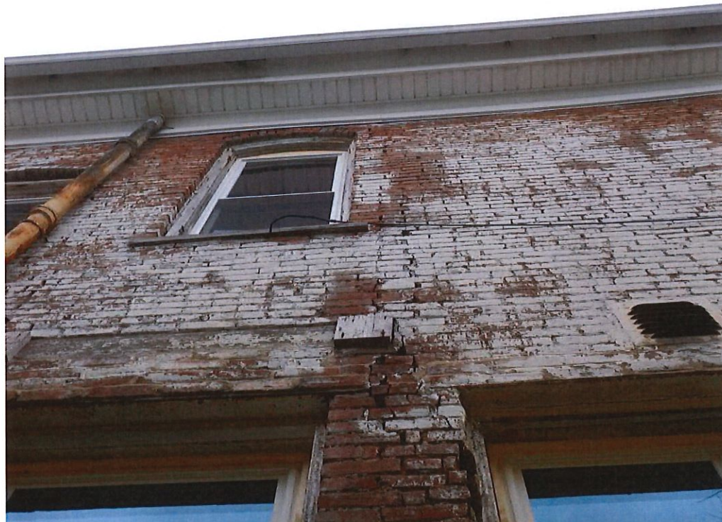
Photo No. 30: Missing mortar and mortar joint cracking on the west side of the building.
