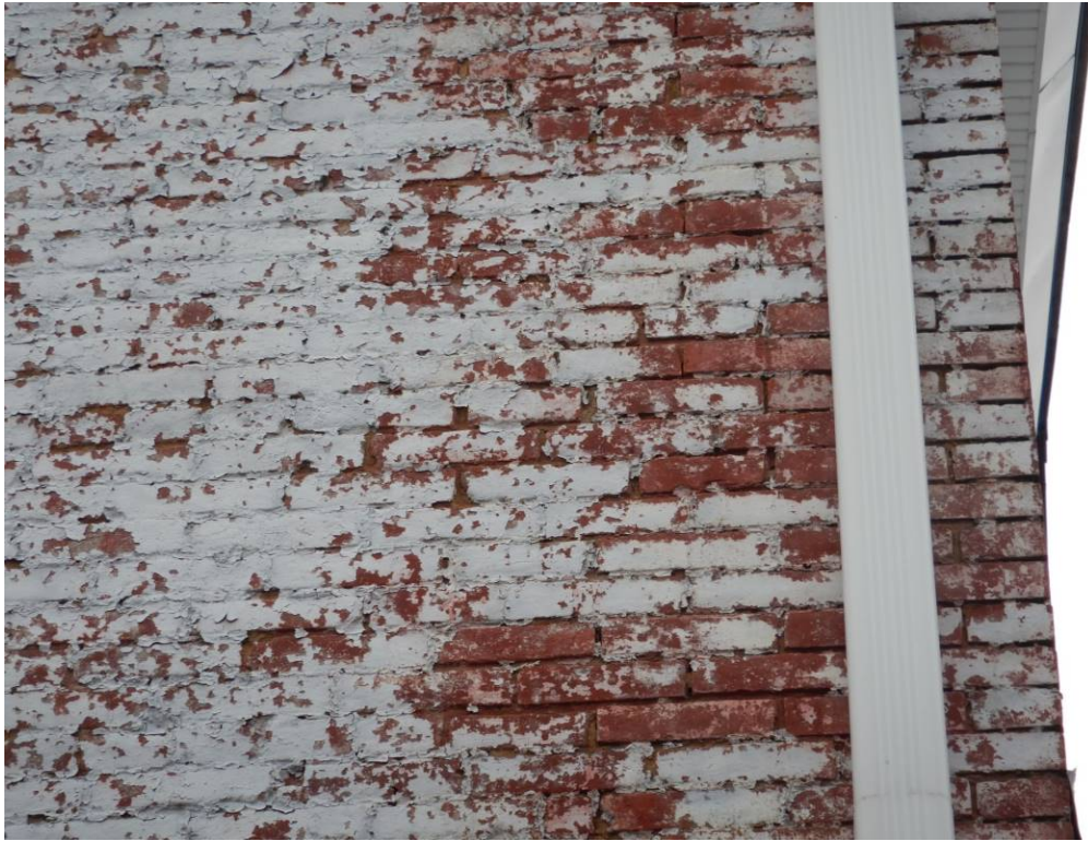
Photo No. 15: Missing mortar and mortar joint cracking on the east side of the building.
