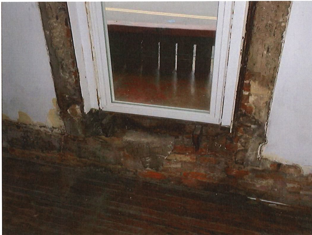
Photo No. 40: Replacement window installation on the main floor with aged water staining.
