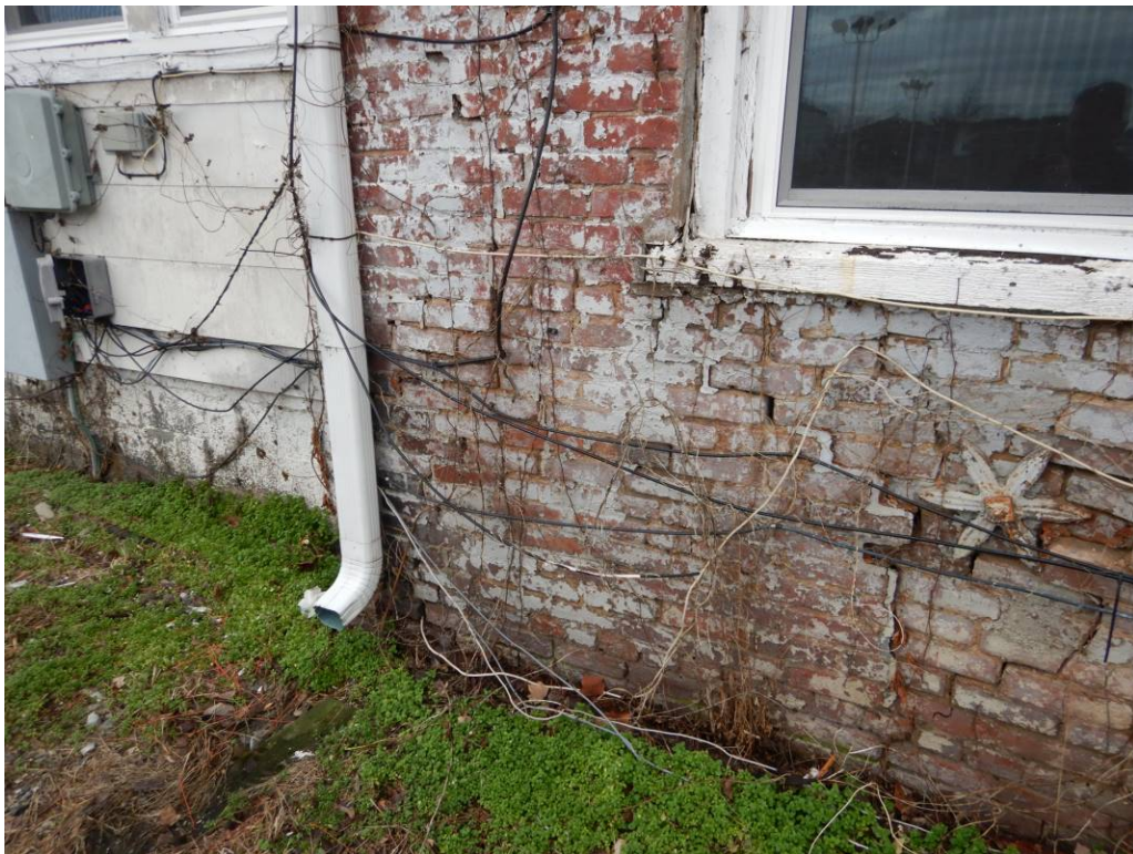
Photo No. 14: Displaced brick masonry on the east side of the building.
