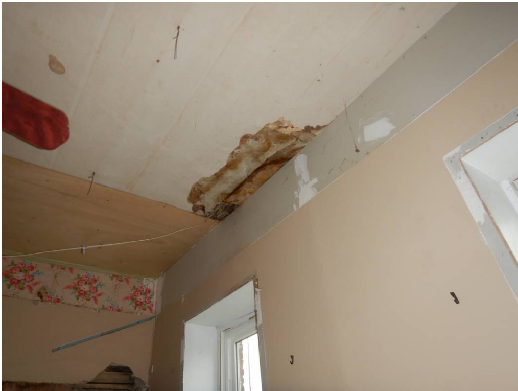
Photo No. 38: Water staining in the ceiling adjacent to a main floor exterior wall.
