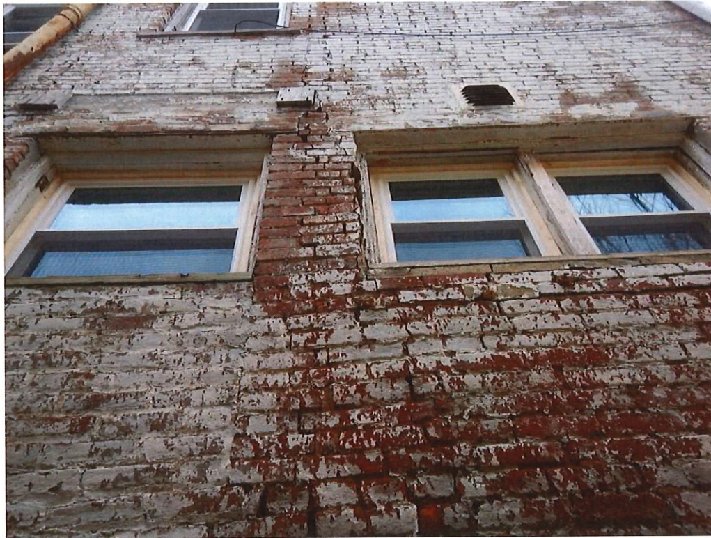
Photo No. 31: Missing mortar and displaced masonry on the west side of the building.
