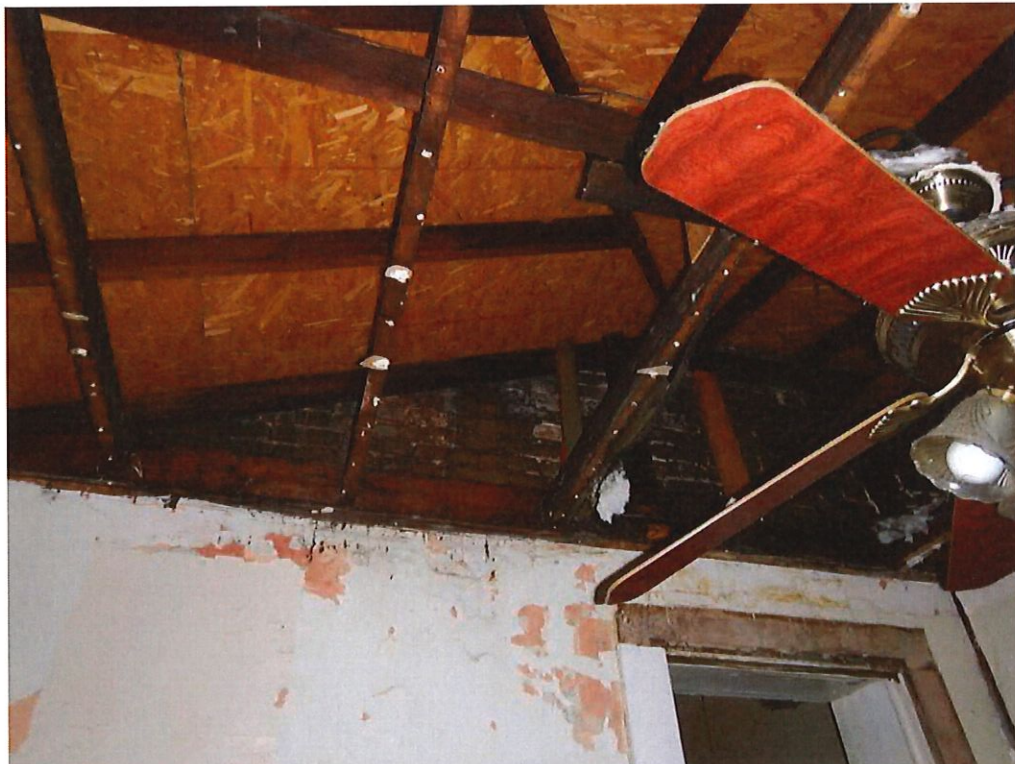
Photo No. 42: Roof structure for the rear addition.
