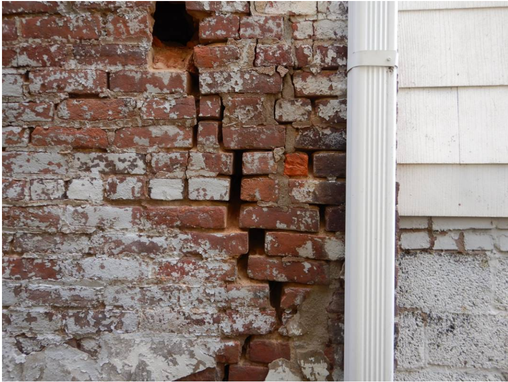
Photo No. 27: Missing mortar and displaced masonry on the west side of the building.
