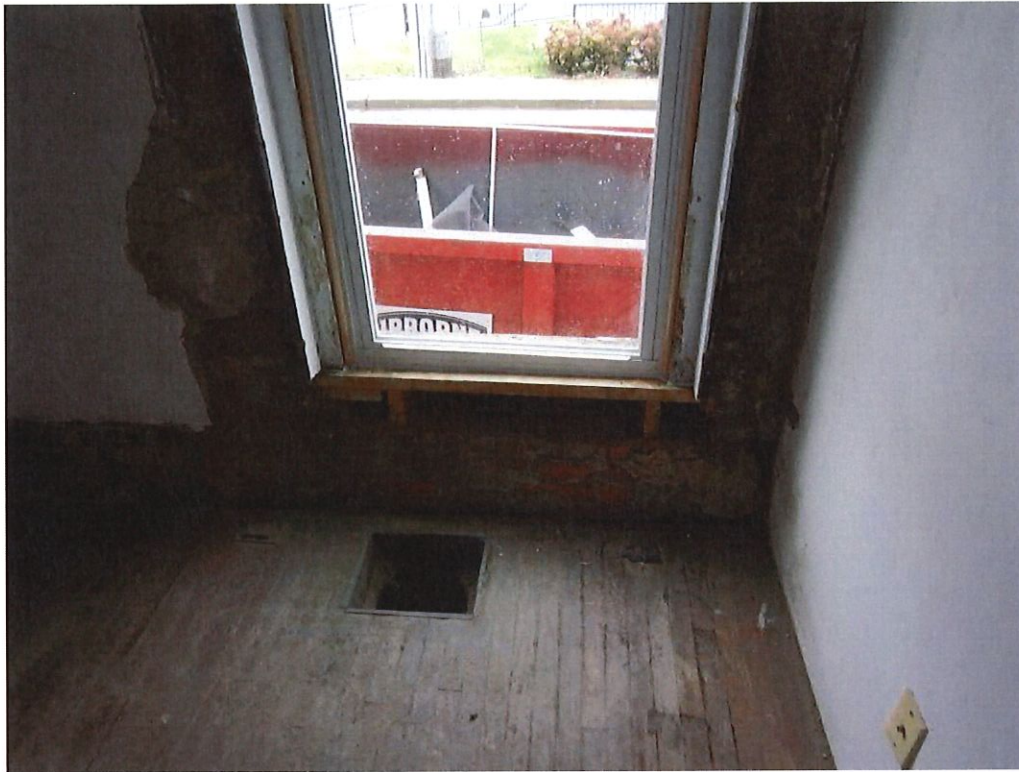
Photo No. 39: Typical replacement window installation on the main floor.
