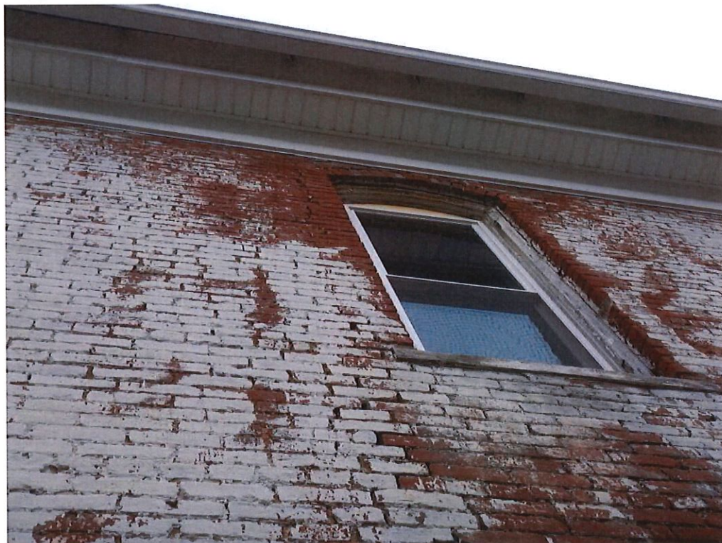
Photo No. 32: Missing mortar and mortar joint cracking on the west side of the building.
