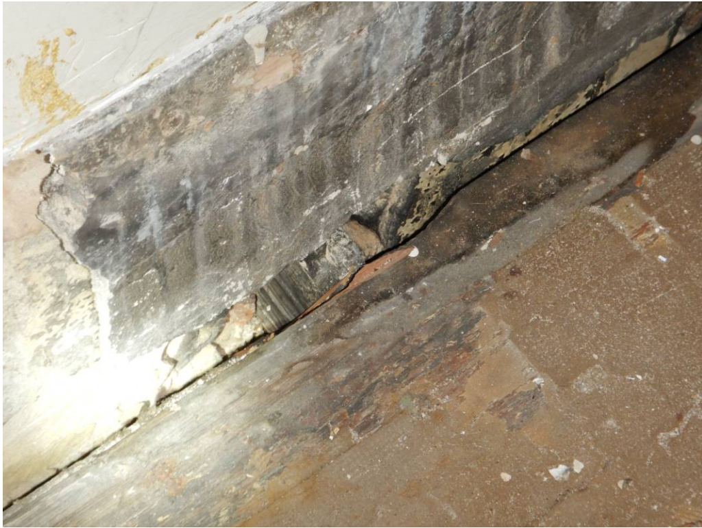
Photo No. 43: Gap between the floor covering and the masonry wall on the upper floor.
