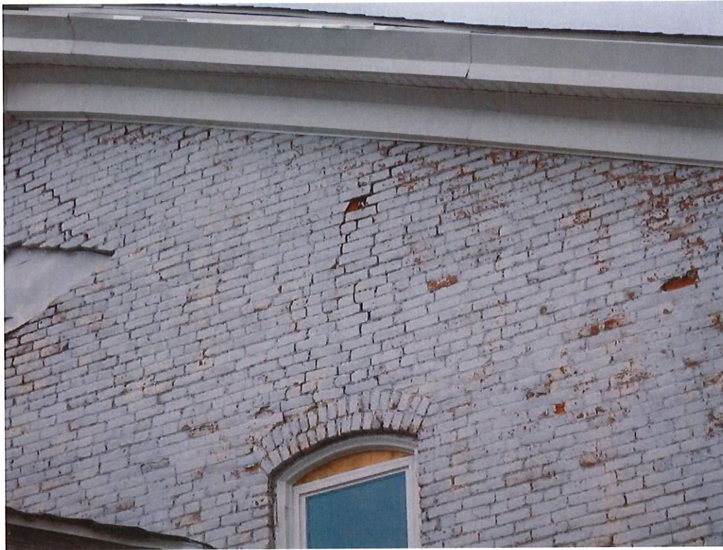
Photo No. 23: Missing mortar and mortar joint cracking on the south side of the building.
