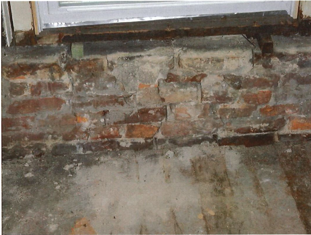
Photo No. 47: Cracked masonry beneath a replacement window installation on the upper floor.
