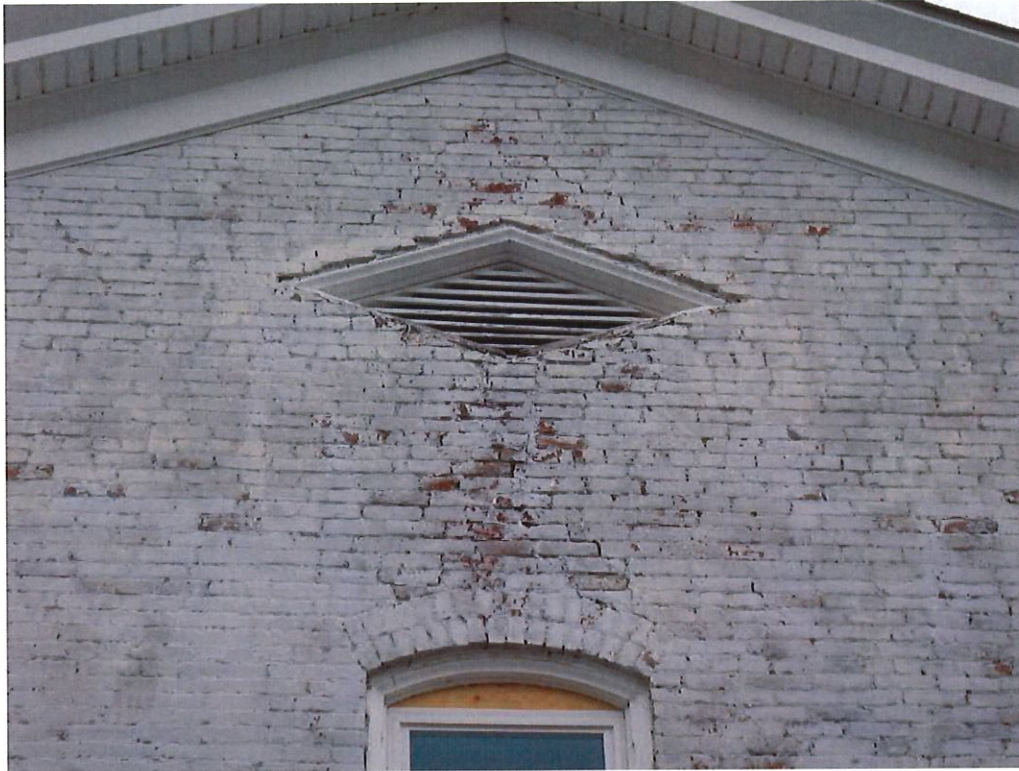
Photo No. 7: Missing mortar and mortar joint cracking on the north side of the building.
