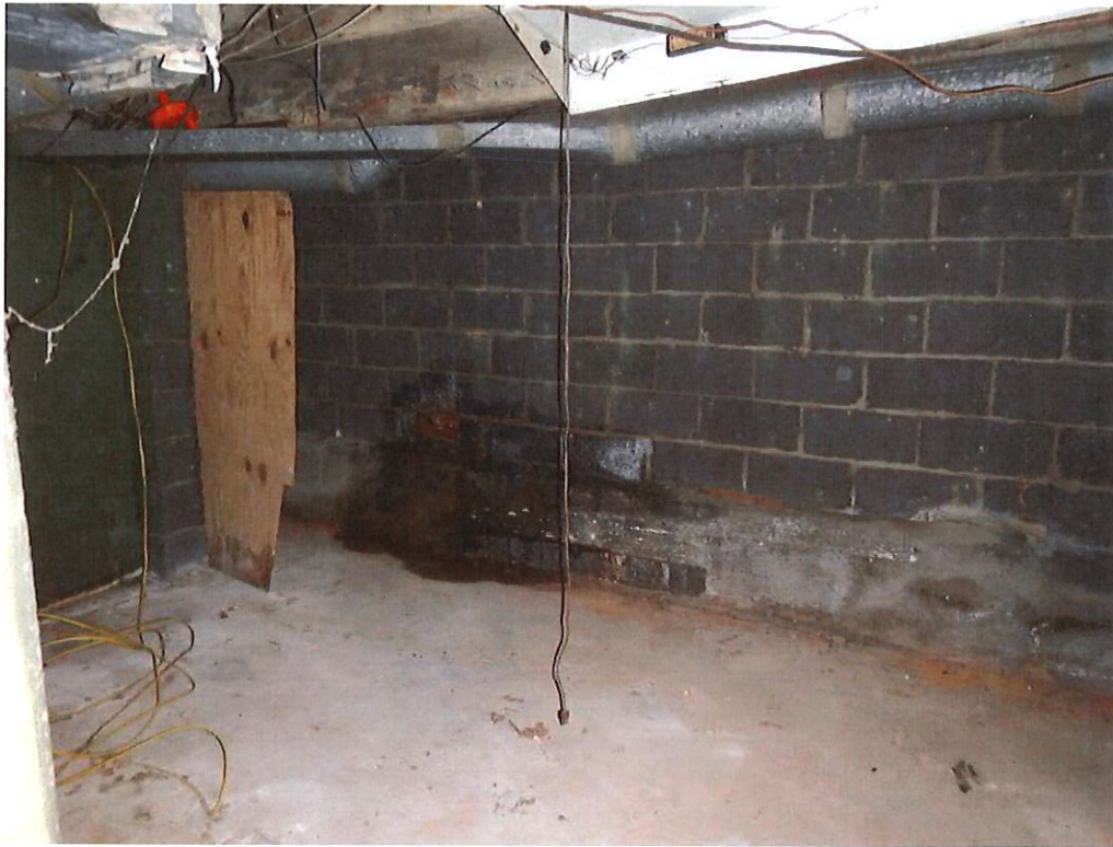
Photo No. 51: Water staining and efflorescence along the base of the foundation wall in the basement.
