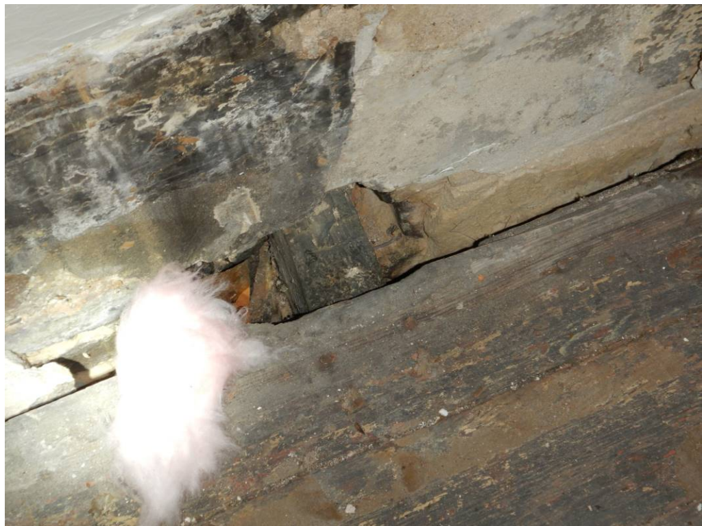
Photo No. 44: Gap between the floor covering and the masonry wall on the upper floor.
