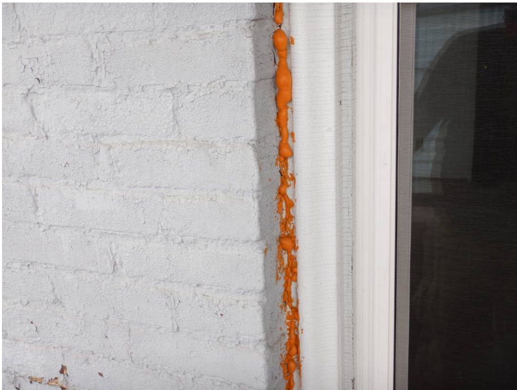
Photo No. 12: Expanding foam sealant along the window trim on the north side of the building.
