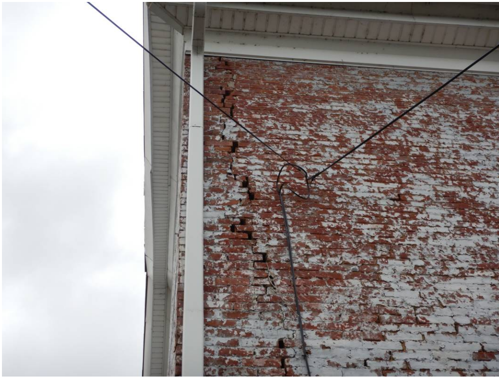
Photo No. 13: Missing mortar and mortar joint cracking on the east side of the building.
