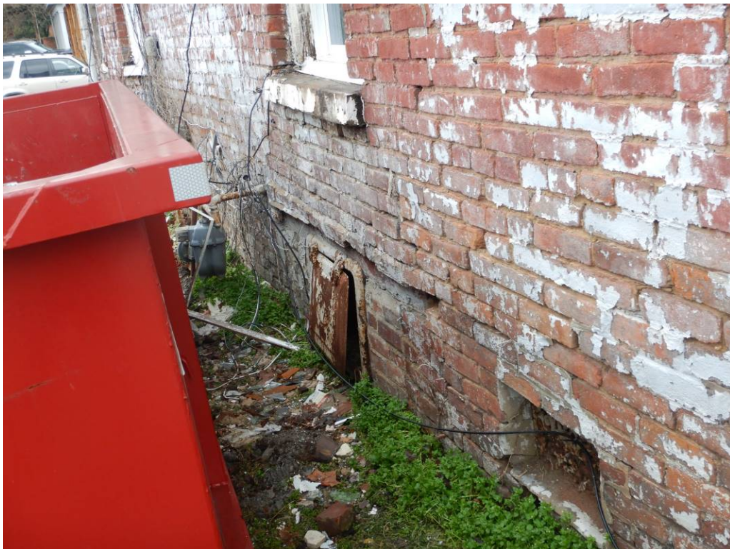
Photo No. 16: Displaced brick masonry on the east side of the building.
