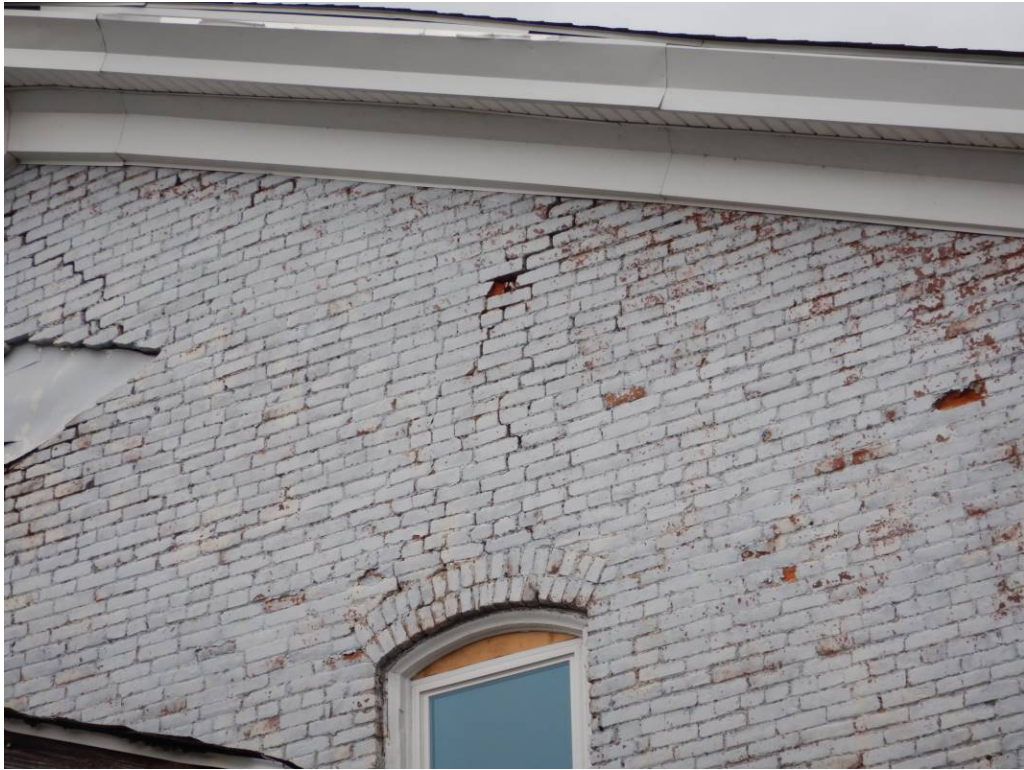
Photo No. 23: Missing mortar and mortar joint cracking on the south side of the building.
