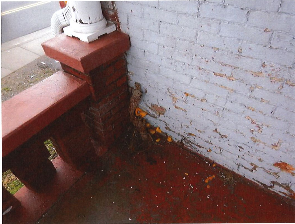
Photo No. 11: Expanding foam sealant and tree growth on the north side of the building.
