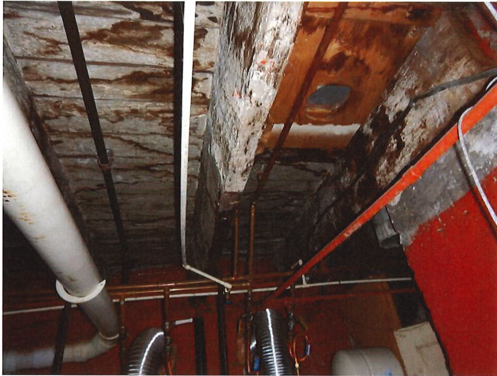
Photo No. 49: Aged water staining on the underside of the main level floor structure.
