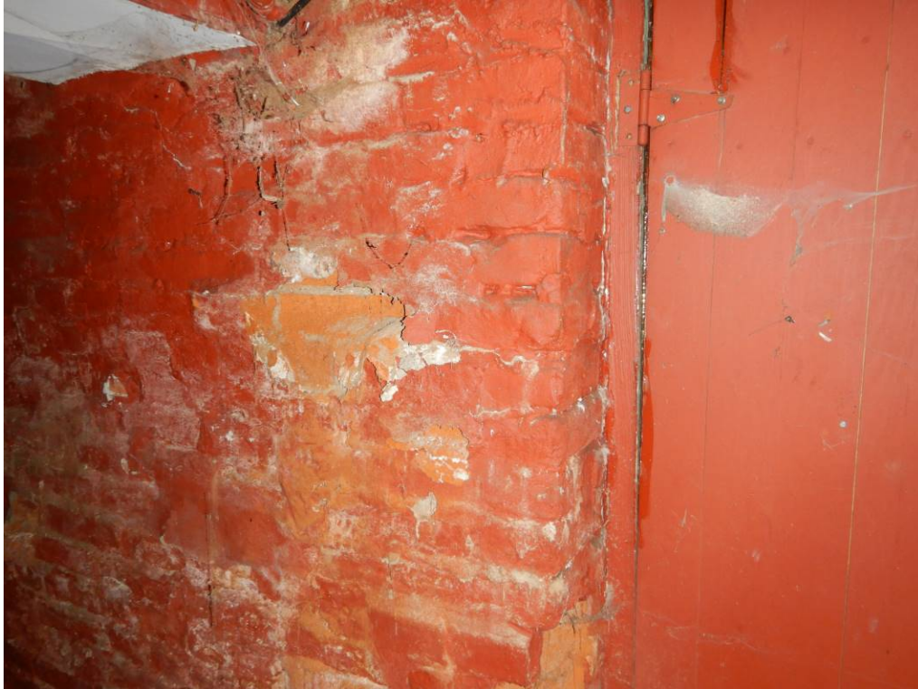
Photo No. 52: Crumbling of mortar and bricks in the basement.
