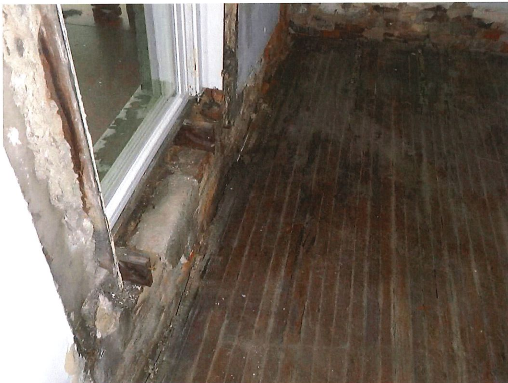
Photo No. 36: Gap between the floor covering and the masonry wall on the main floor.
