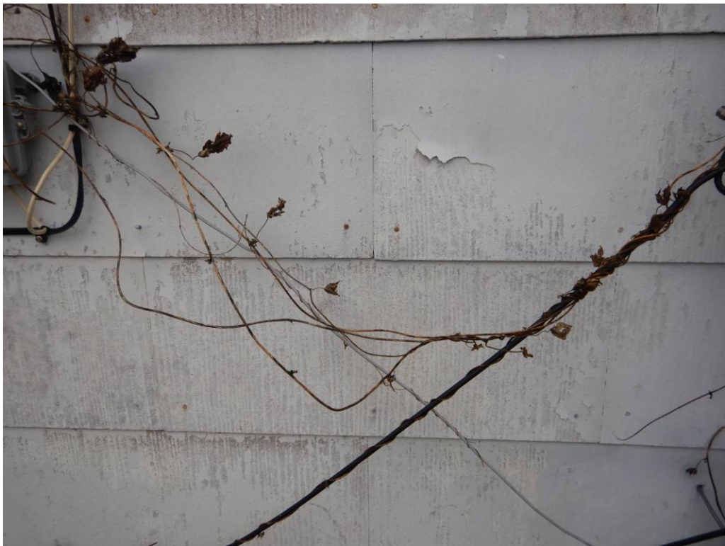
Photo No. 24: Asbestos siding on the rear addition on the south side of the building.
