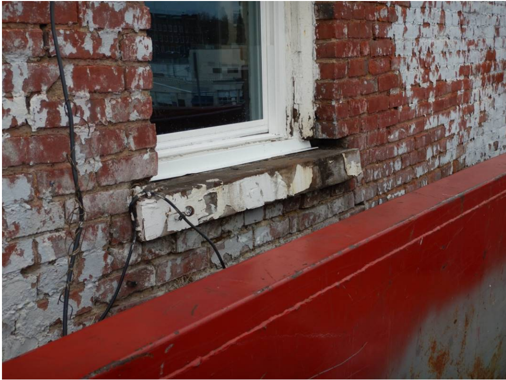
Photo No. 17: Displaced window sill on the east side of the building.
