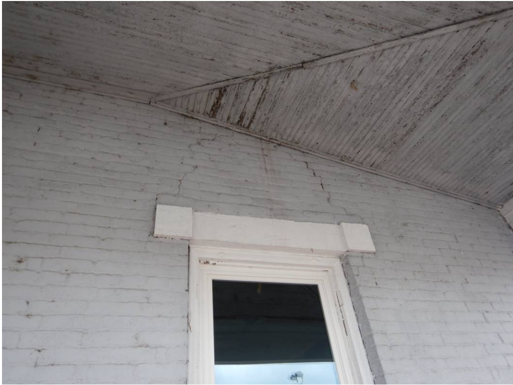
Photo No. 9: Missing mortar and mortar joint cracking on the north side of the building.
