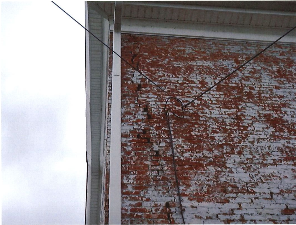
Photo No. 13: Missing mortar and mortar joint cracking on the east side of the building.
