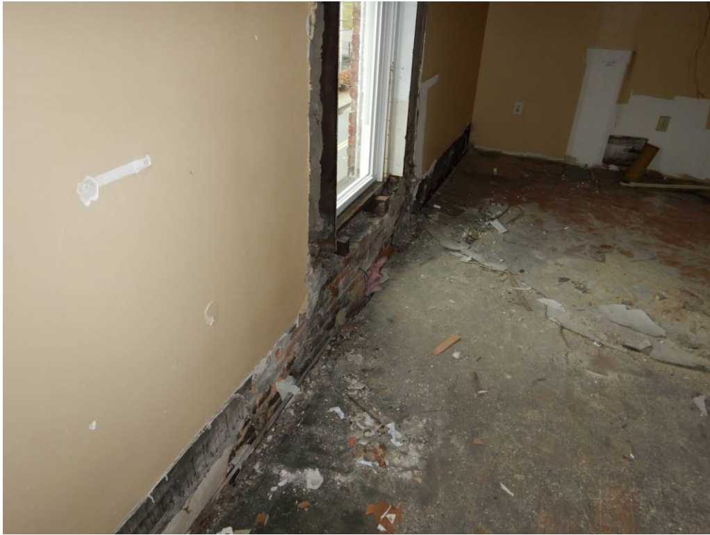
Photo No. 45: Gap between the floor covering and the masonry wall on the upper floor.
