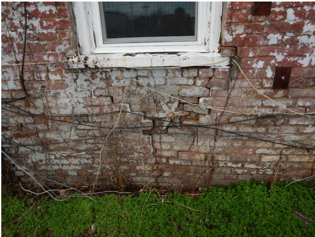
Photo No. 18: Displaced brick masonry on the east side of the building.
