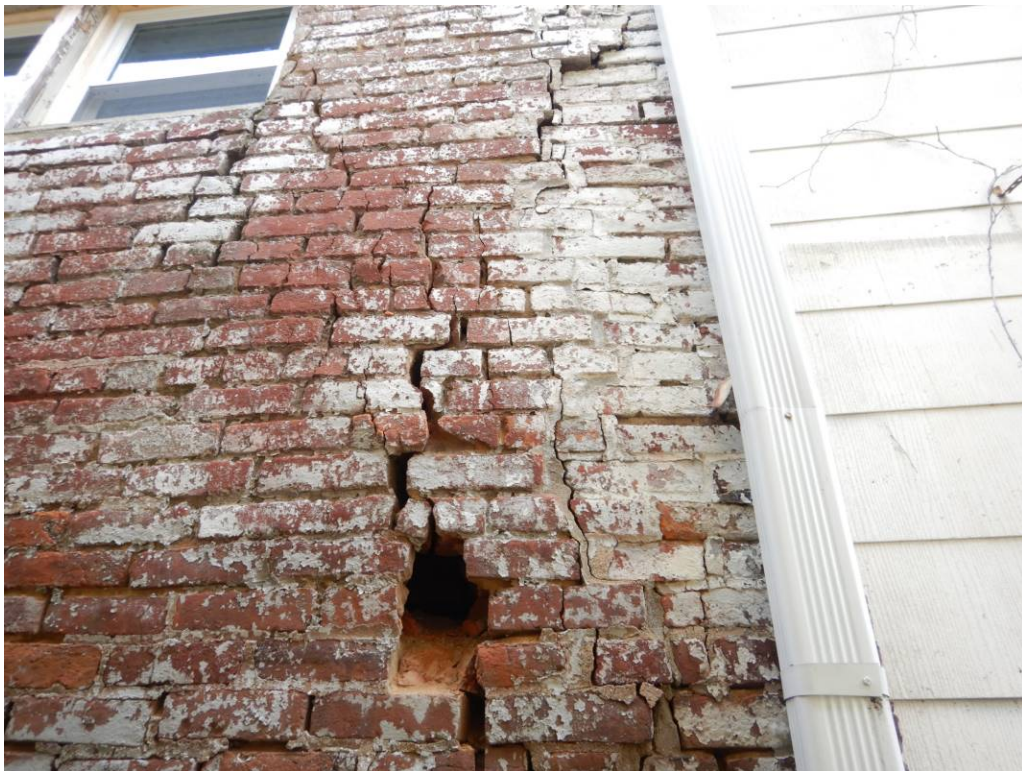
Photo No. 26: Missing mortar and displaced masonry on the west side of the building.
