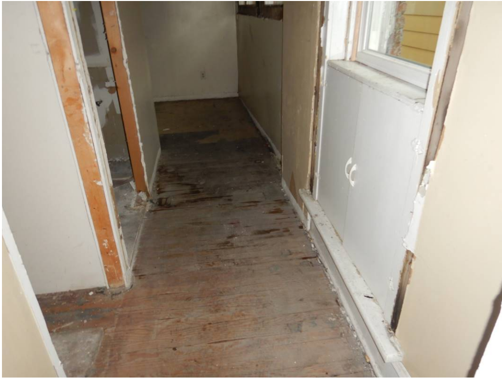
Photo No. 35: West wall bowed away from the floor structure on the main floor.
