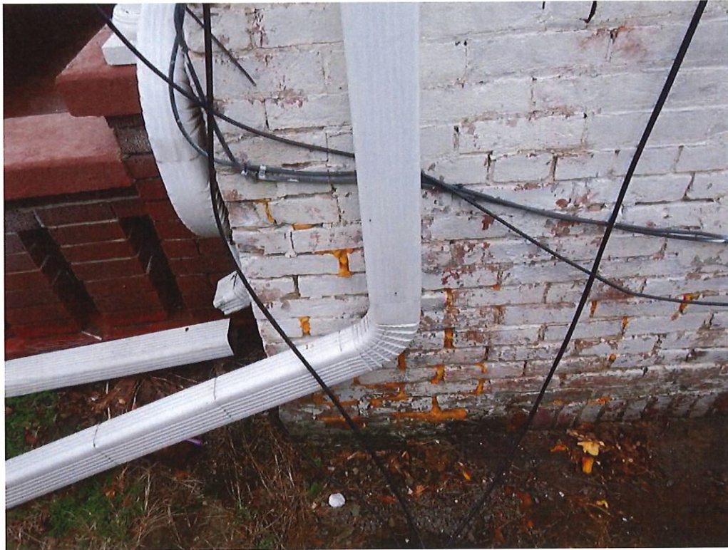
Photo No. 33: Expanding foam in locations of missing mortar.
