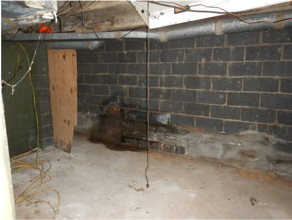
Photo No. 51: Water staining and efflorescence along the base of the foundation wall in the basement.
